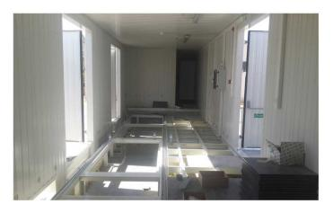
Depending on the continuous technical support from Schneider Electric to our crew, and the using of its products, Al-Handasys has presented its own designs for mobile substations distributed on two trailers, to be connected together on site, to form an integrated unit.
