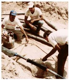
The cross-linking process results in an "elastic memory", activated simply by heating. The memory then causes the components to shrink to a predetermined diameter; the correct insulation thickness is thus achieved in one step automatically.
