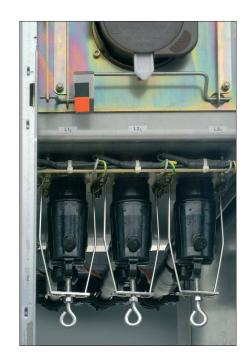
In addition, Rayvolve tubing or heatshrink phase-marking sleeves are offered as an option, to provide a superior environmental seal.
